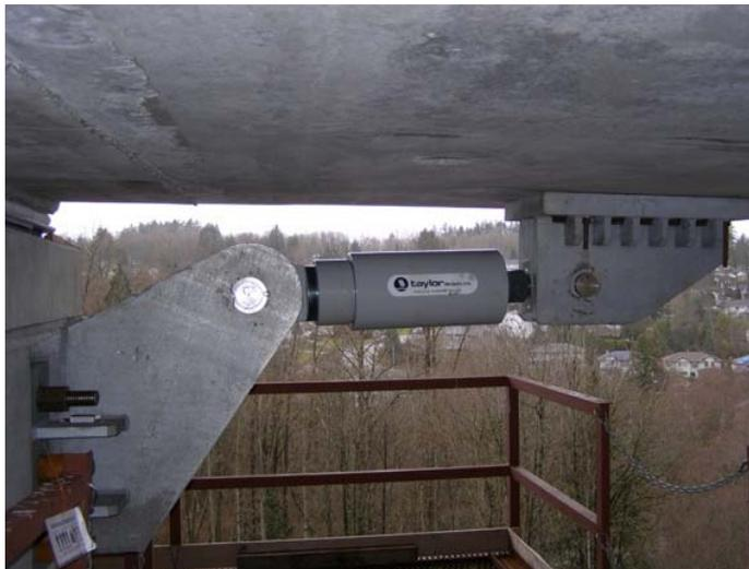
Seismic Protection using 146 Taylor Device
